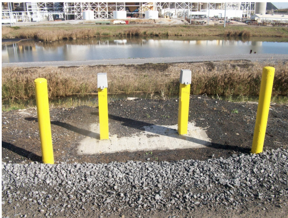
Figure 5. Typical Instrumentation (Slope Inclinometers, Piezometers) Installation
