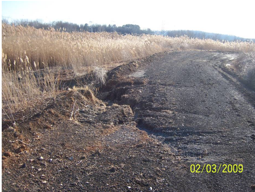
Drawing Mark DS-1-5 Erosion and rutting along access road at the base of the Dry Ash Stack.
