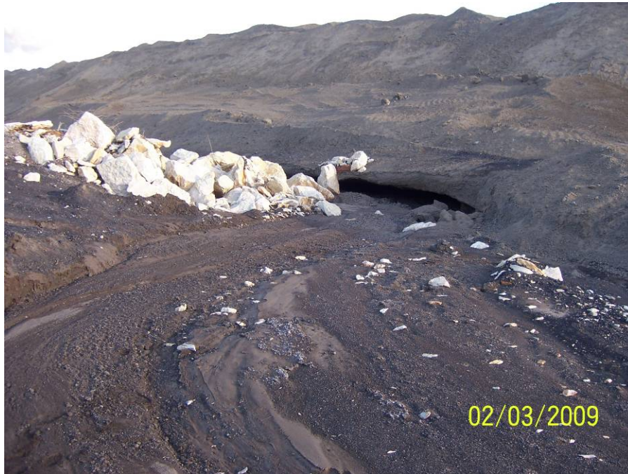
Drawing Mark DS-1-3 Erosion around existing rock check in north portion of Dry Ash Stack
