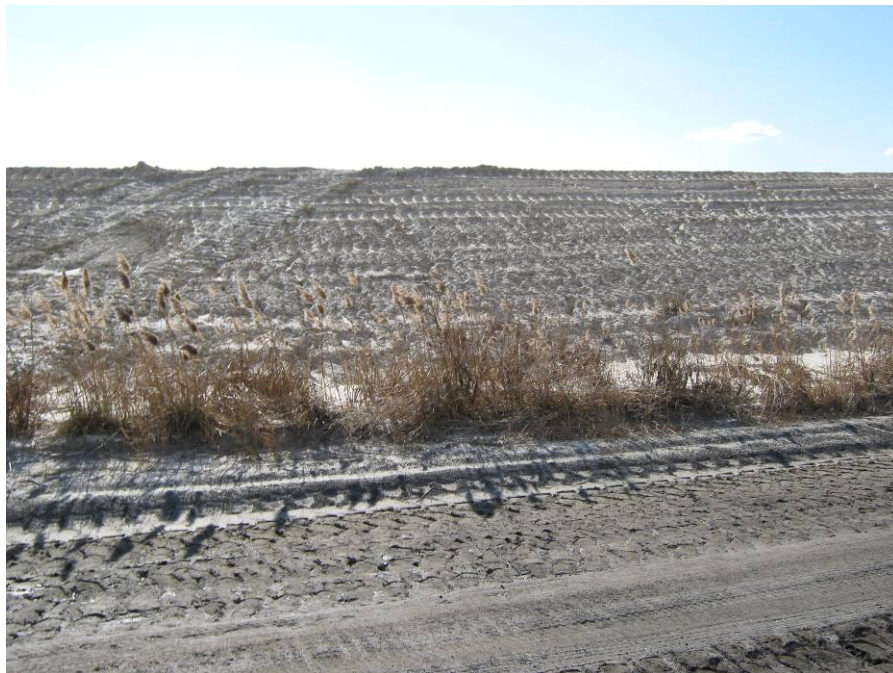
Drawing Mark GP-1-4 Reconstructed gypsum dikes surrounding the two ponds lacking vegetation.
