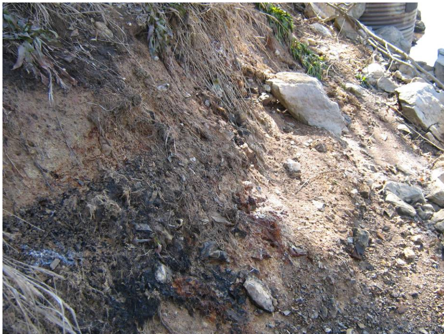
Drawing Mark DS-1-2 Seepage observed below the perimeter dike along the banks of Wells Creek.
