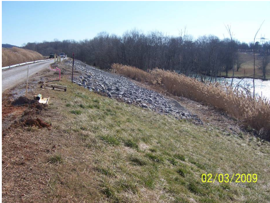
Drawing Mark GP-1-1 Riprap placed in area to temporarily repair slope slough along the perimeter dike at the NW corner of the Gypsum Stack.
